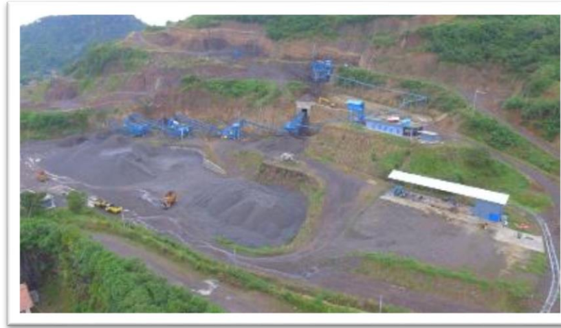
QUARRY & CRUSHING PLANT
