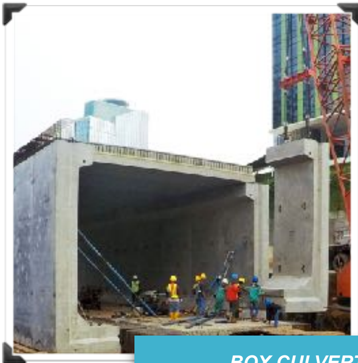
BOX CULVERT DEPOK-ANTASARI TOLL ROAD
