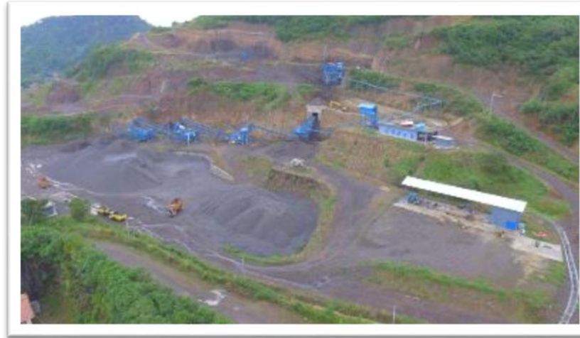
QUARRY & CRUSHING PLANT
