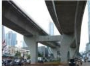
Overpass Kamp. Melayu – Tanah Abang (2014)
