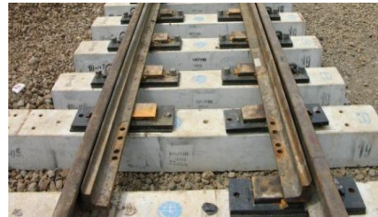
KA-Clips, DE-Clips, Pandrol, E-Clips, and Vossloch
