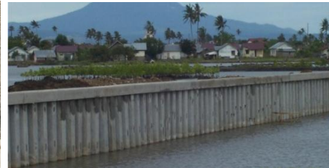
Corrugated concrete (CCSP) dan Flat sheet piles (FCSP).
