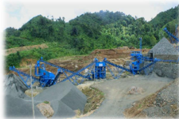
QUARRY & CRUSHING PLANT
