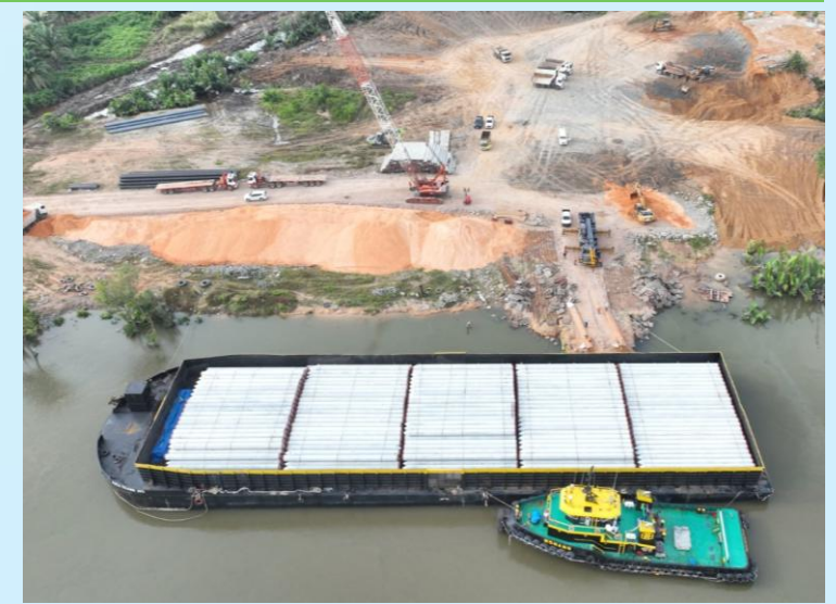
Shoring Protection Area Shiploader Tanah Grogot, Kalimantan Timur
